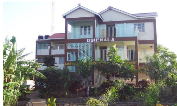
Figure 2: Front view of the Research Center at Dunga Beach Kisumu
